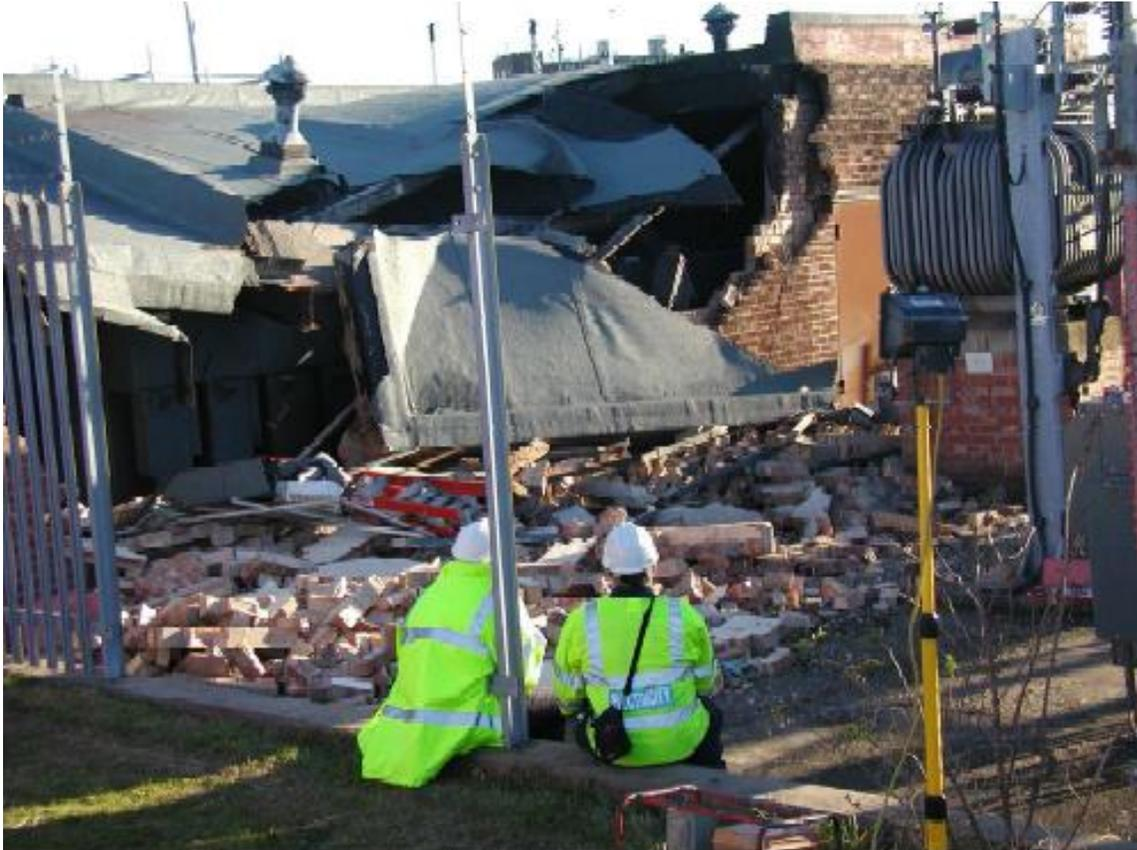
**Figure 1 Damage to substation following a catastrophic switchgear failure**
