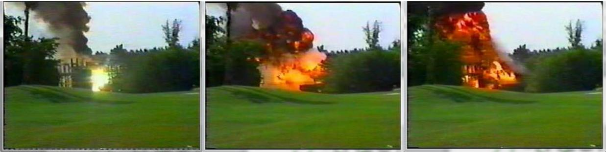
**This FPL substation (138KV stepped down to 23KV) adjacent to a Miami golf course and residential community was a total loss in just minutes. <http://205.243.100.155/frames/longarc.htm#Disconnect>**
