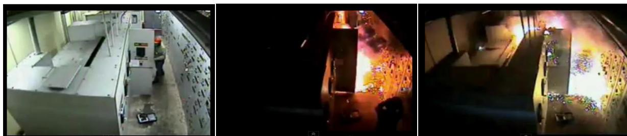
**Arc Flash while racking a breaker in MV switchgear; location and worker injury unknown.**
